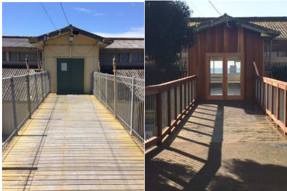
The old façade (left) & the new façade (right)
